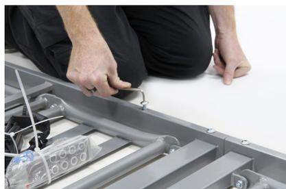
Once the platform sections are together install the final fixing screws.
